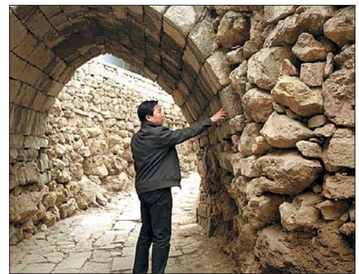
The Qing Dynasty single-arched stone-made bridge is composed of two levels of roads, one on top of the other.
